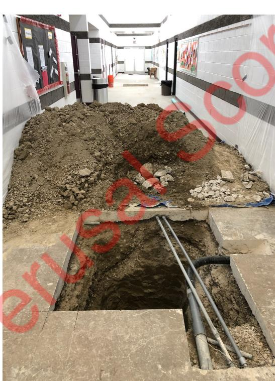
(It turns out workers had to cut into the floor and dig down to repair a broken pipe.)
